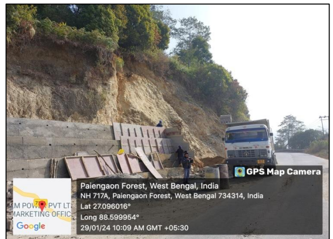
Structural measures taken to protect landslide areas, Algarah and its surroundings, Kalimpong district, West Bengal
